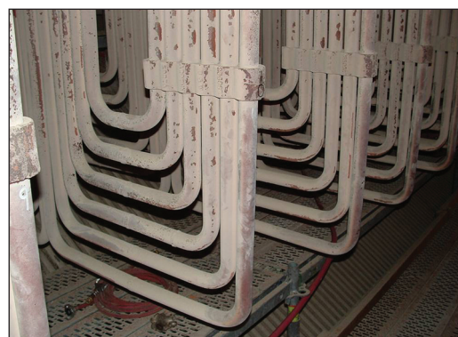
Figure 8: Superheater assemblies.
