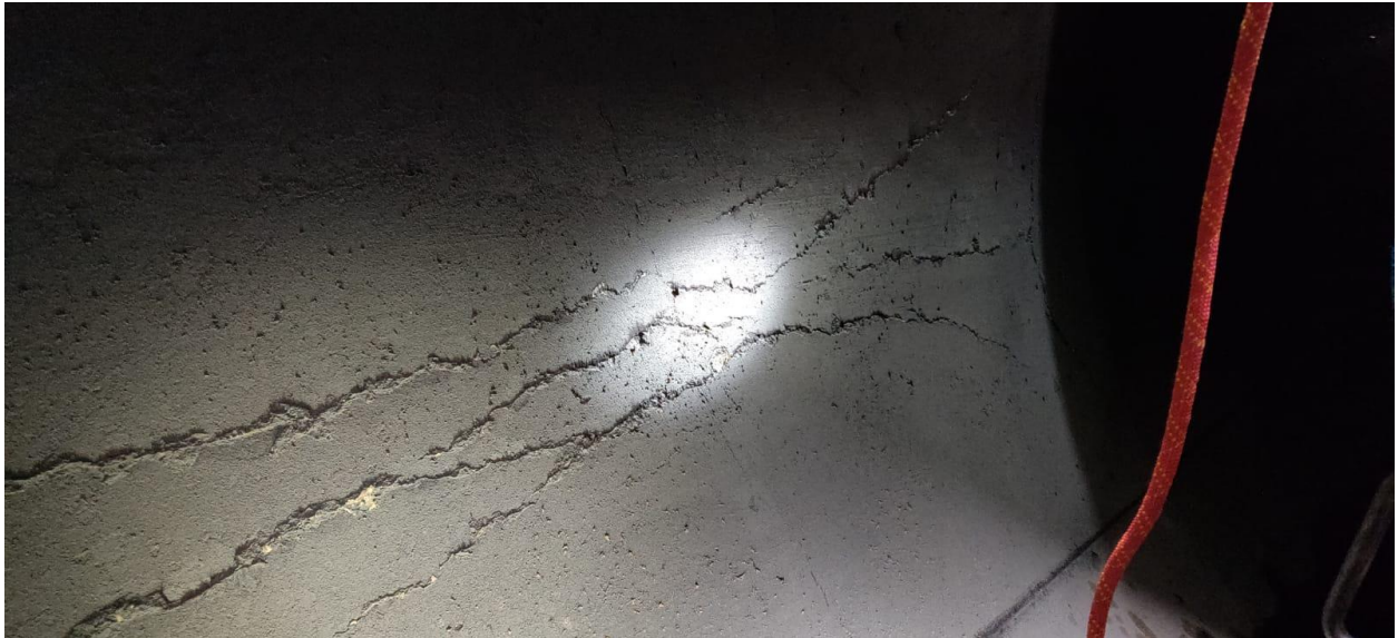
Axial Cracking on the concrete line pipe
