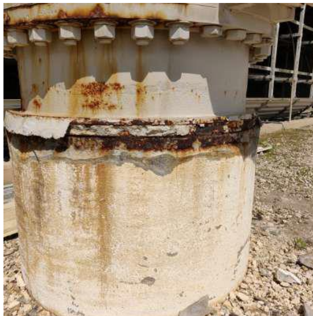
Mortar Coating failure on Riser B
