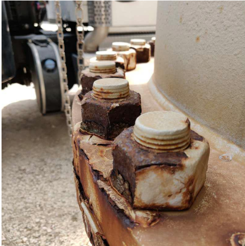
Severe bolt corrosion on flange
