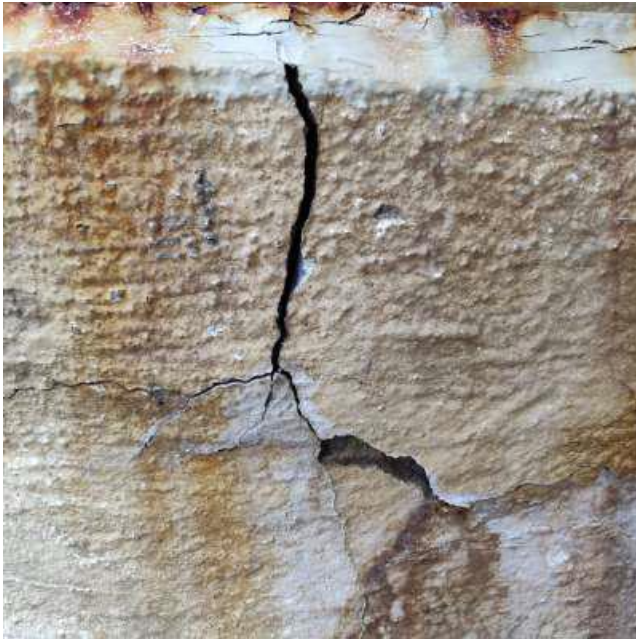
Deep Mortar Cracks on a Riser Pipe
