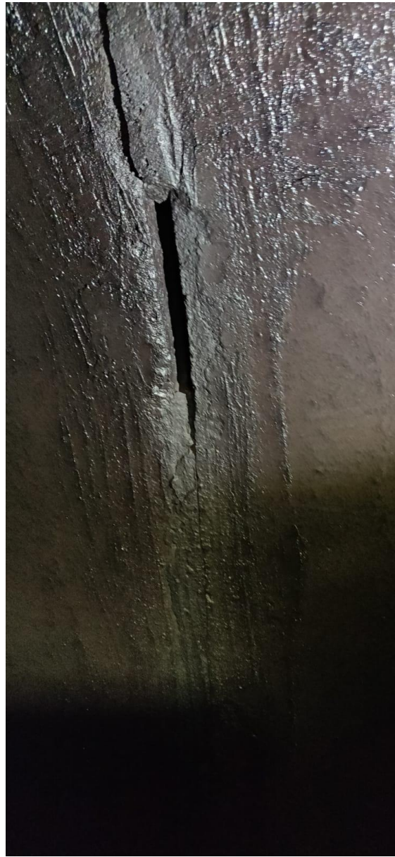
Concrete Gap at Joint
