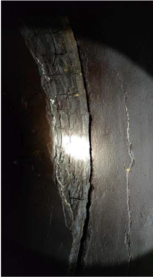
Cement Disintegration
