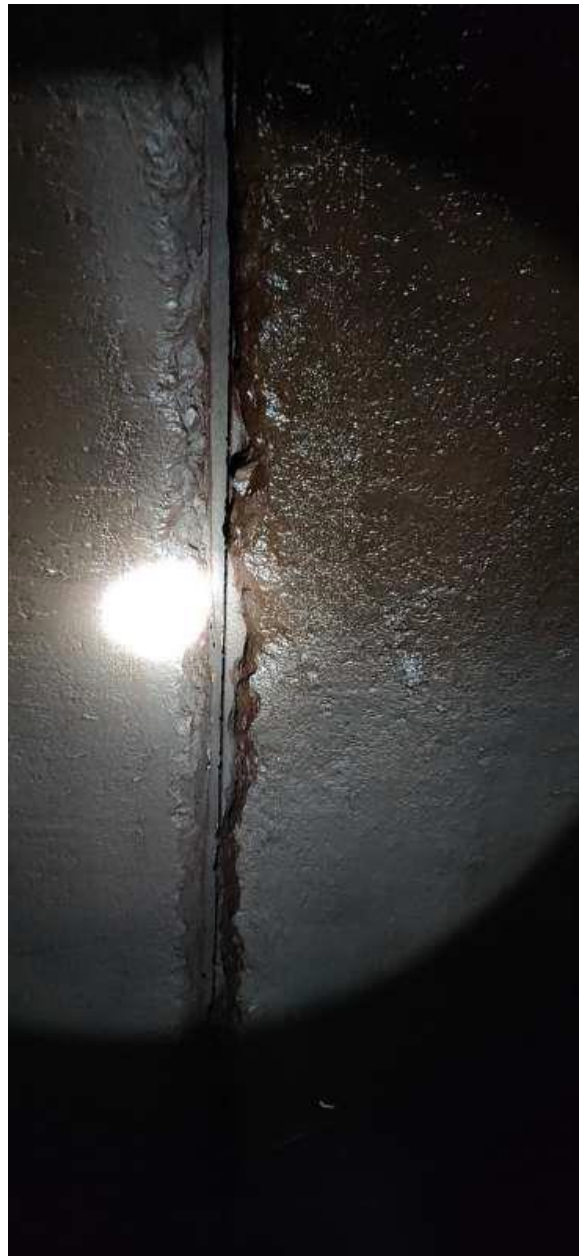
Cement Gap at a Joint
