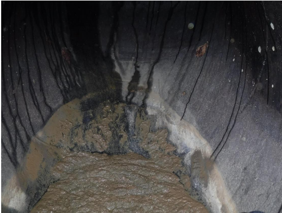
Excessive amount of mud found in Circulating Water Line.
