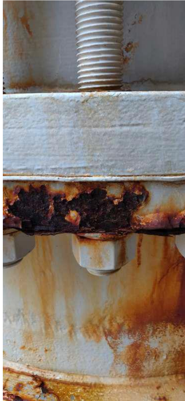
Corrosion Deterioration at flange
