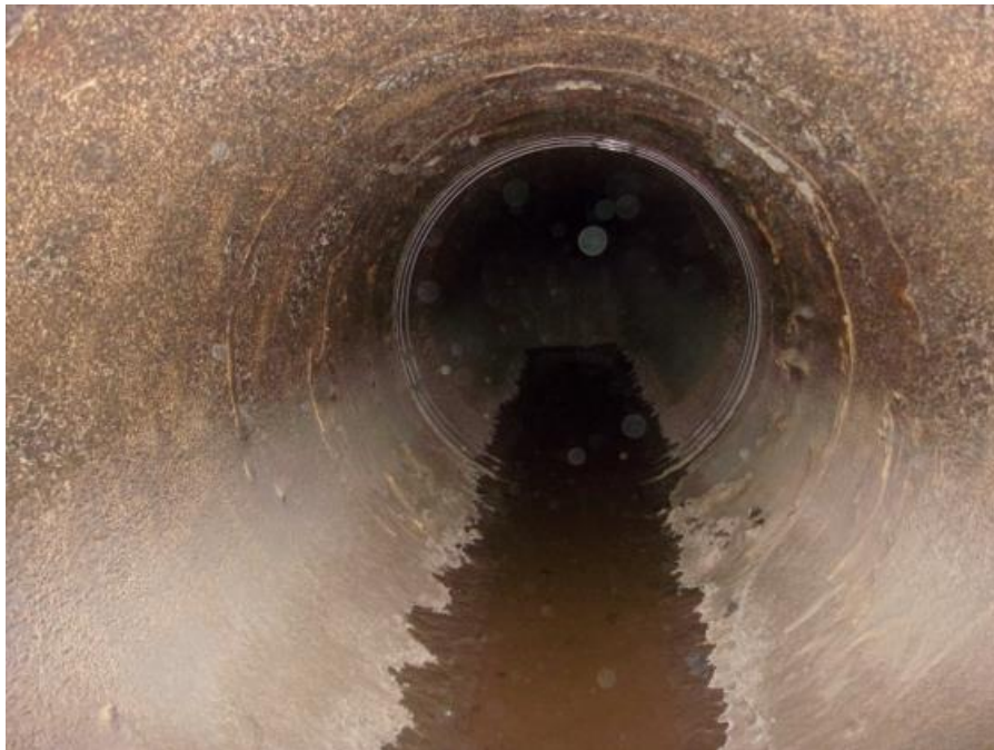
Circulating Water Line showing the concrete surface with coating in some areas
