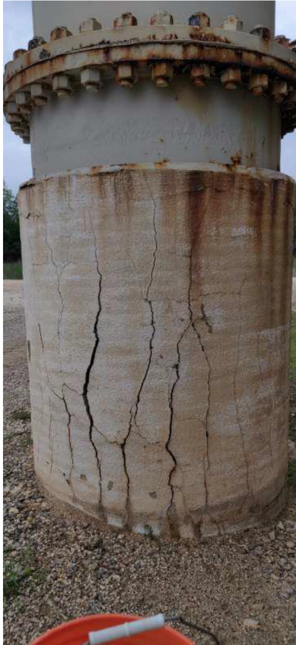
Deep Cracks in the Mortar coating on a Riser Pipe
