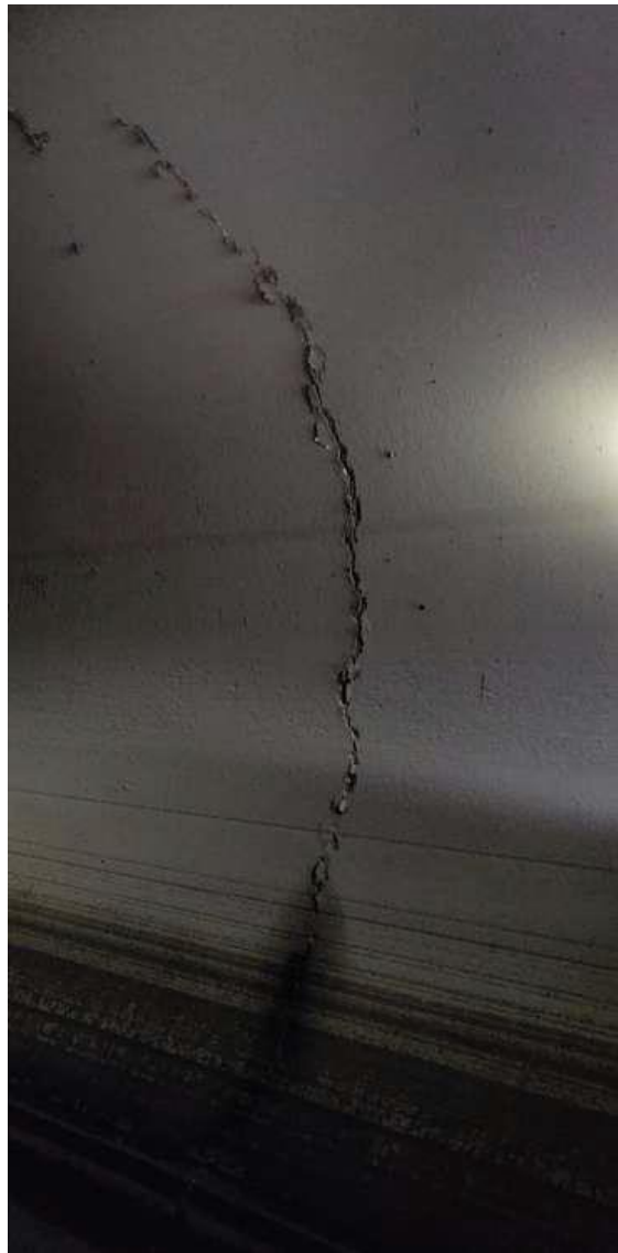
Circumferential Crack between joint 1 & 2
