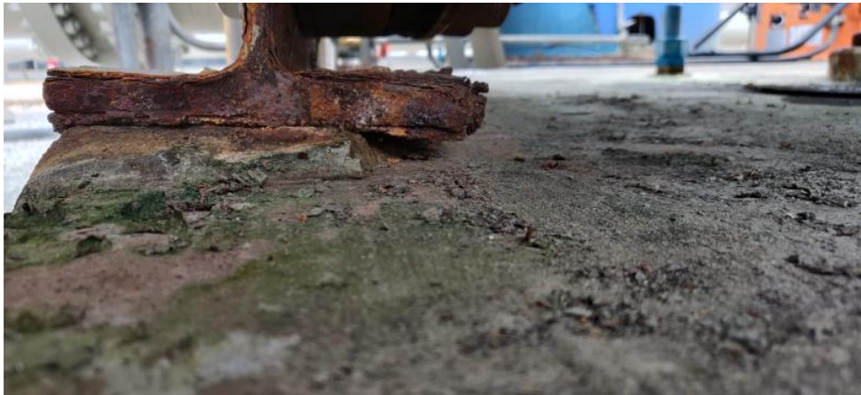
Side view of I-beam support with active corrosion
