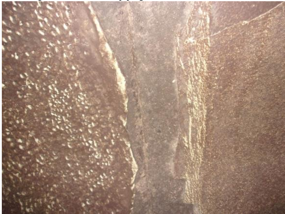
Coating Failure at a concrete joint
