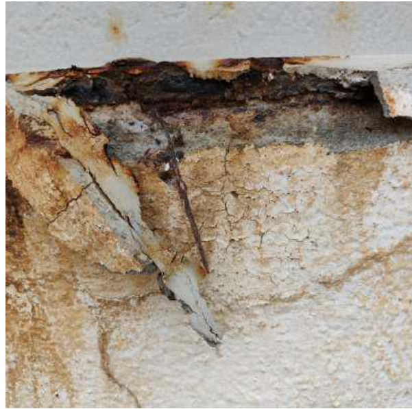
Prestressed wire exposed and broken on mortar coating of a Riser Pipe
