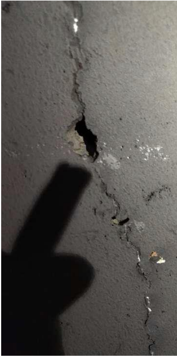
Cracking and Pitting on concrete liner
