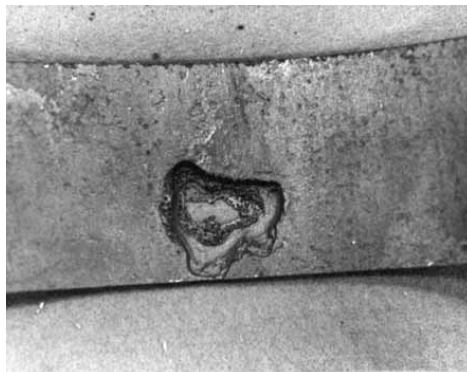
Figure 2. Microbiologically induced corrosion pits often have a terraced effect.
