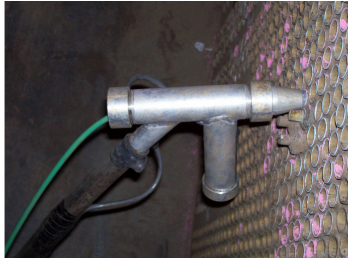
Figure 3 shows the air assist gun as a probe is ready to shoot through the condenser tube.
