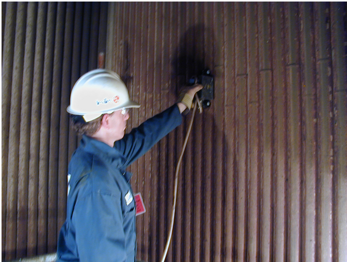
Figure 3 shows a LFET Inspection being performed on a water wall
